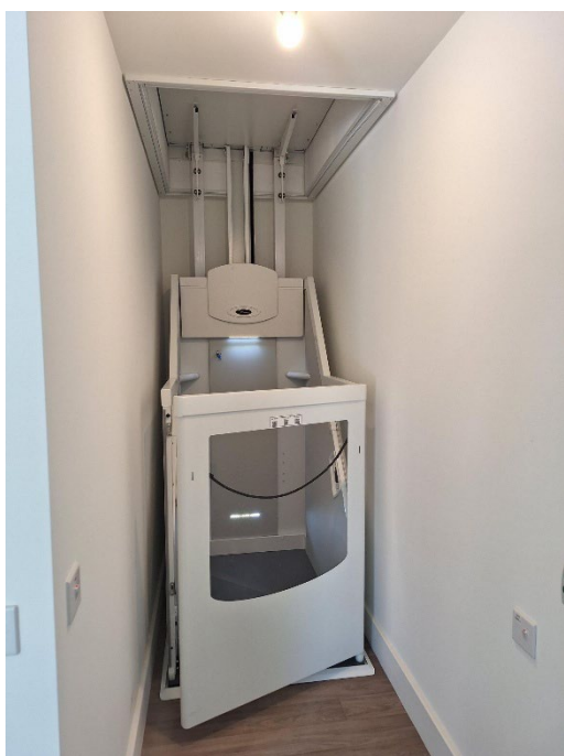
Picture 4: Photo showing the through-floor lift installed in the purpose-built, fully accessible home at Woodlands Place.
